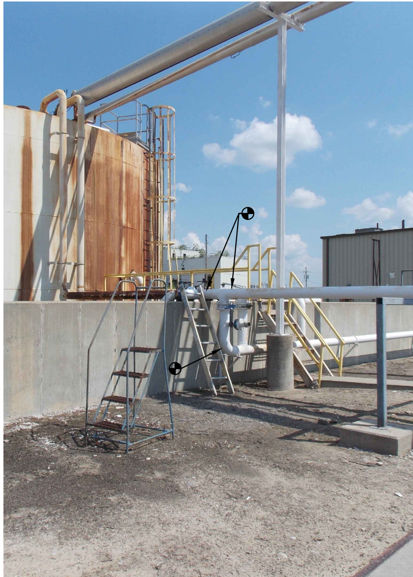
Photo O Connection Location for Diversion of Pumped Waste.
