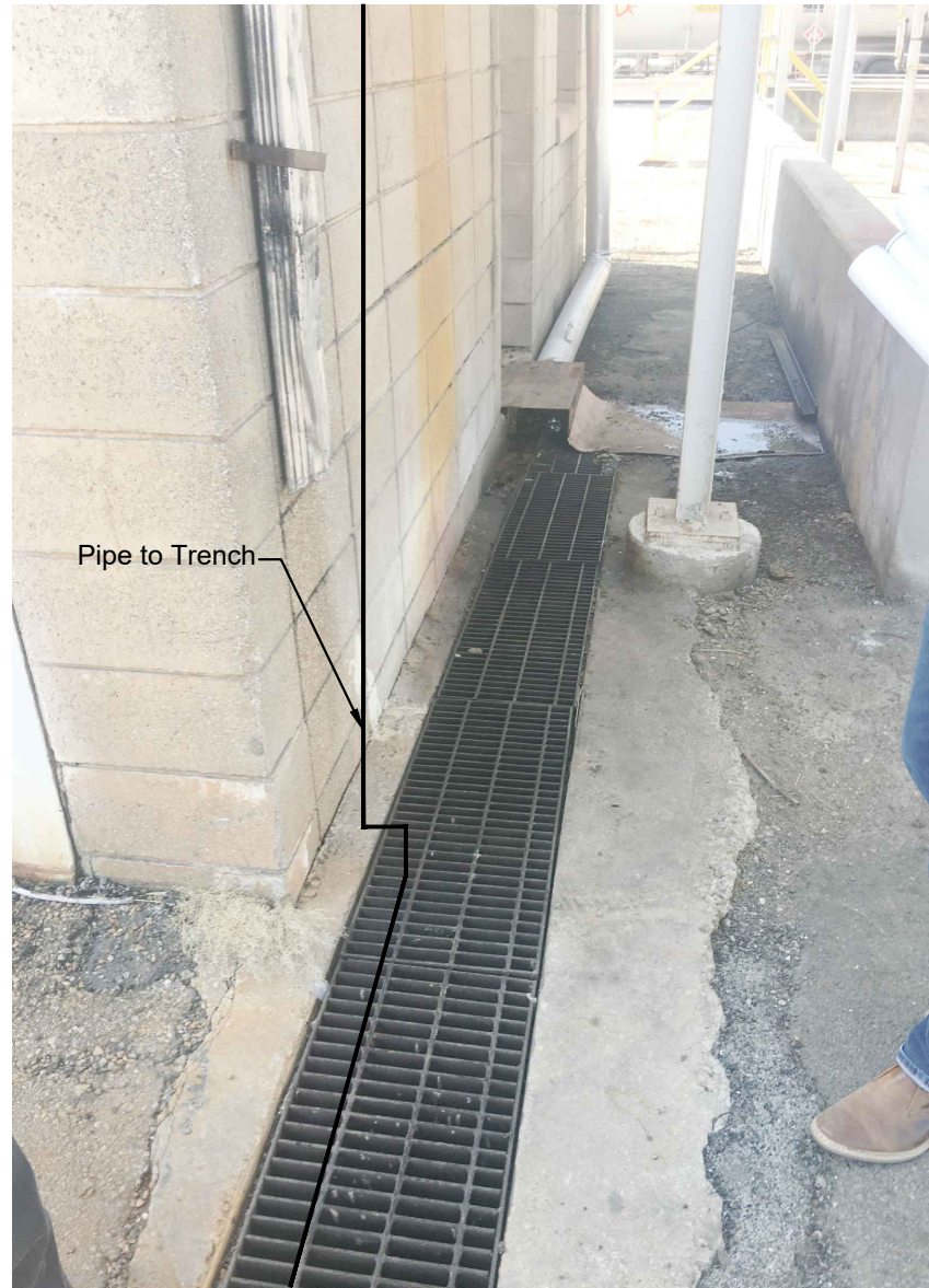
Photo I Route Pumped Waste under Open Grate to Catch Basin.
