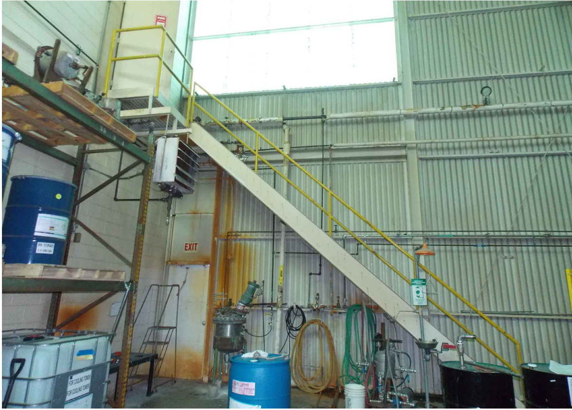
Photo C Penetration location for pumped waste from Air Operated Diaphragm Pump.
