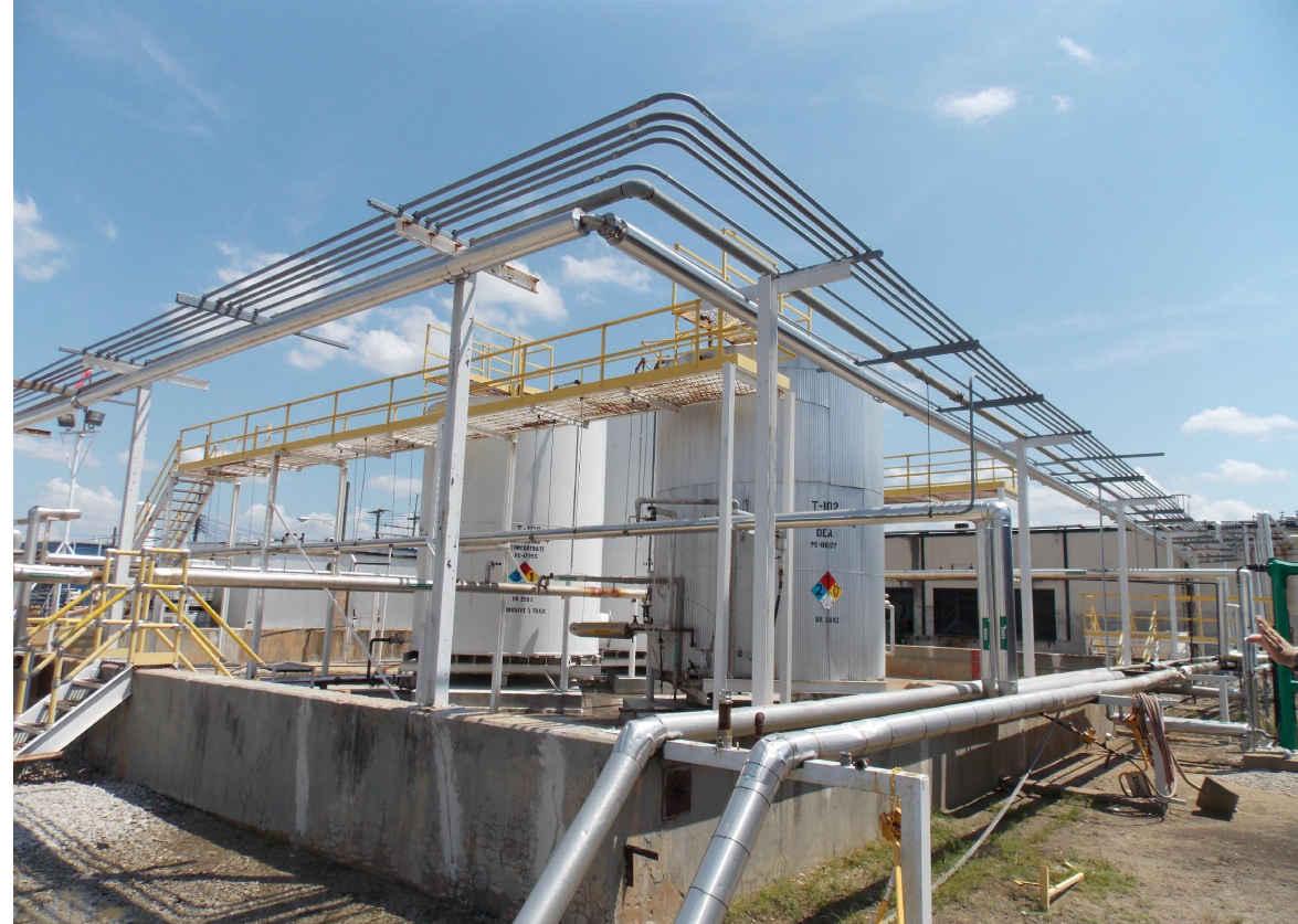
Photo G Pumped Waste Routing on Existing Pipe Stands.
