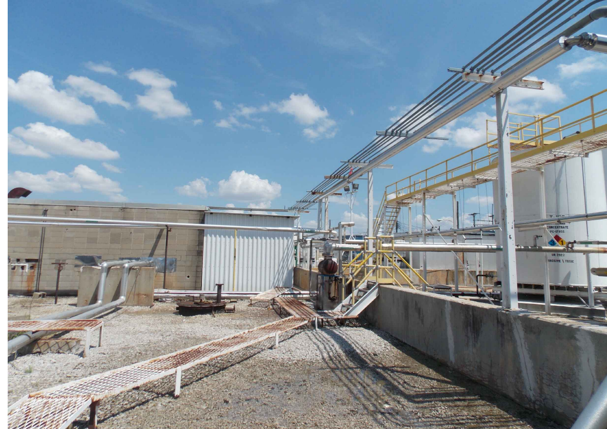
Photo H Pumped Waste Routing on Existing Pipe Stands.
