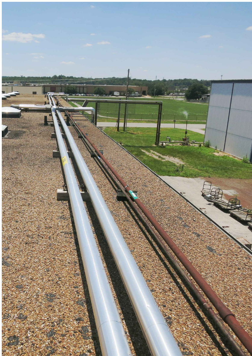
Photo F Formulation Building Roof. Provide Roof Blocks for New 2" Compressed Air, 2" Nitrogen, and 4" Pumped Waste.
