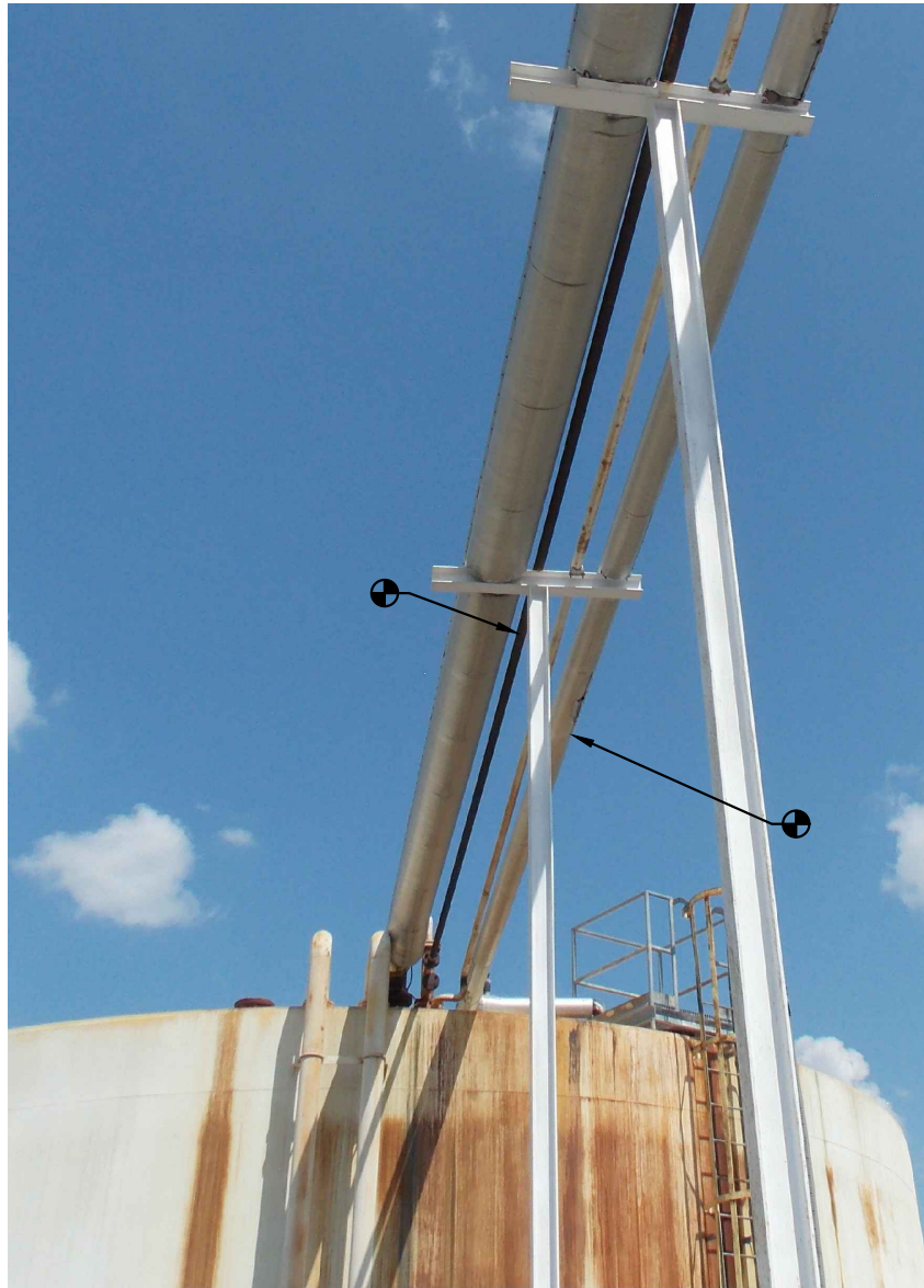
Photo N Connection Location for Diversion of Scrubber Tank Discharge and Emergency Retention Basin Discharge.
