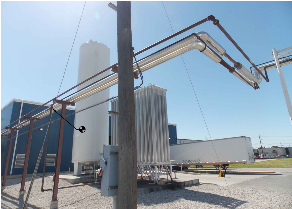
Photo J Connection Location for 2" Nitrogen.
