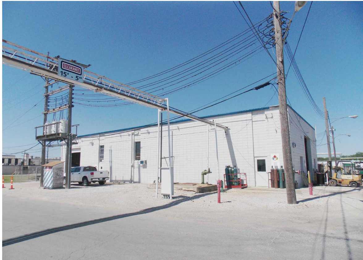
Photo K Existing Pipe Bridge for Routing of 2" Nitrogen. Route Over Existing Building.
