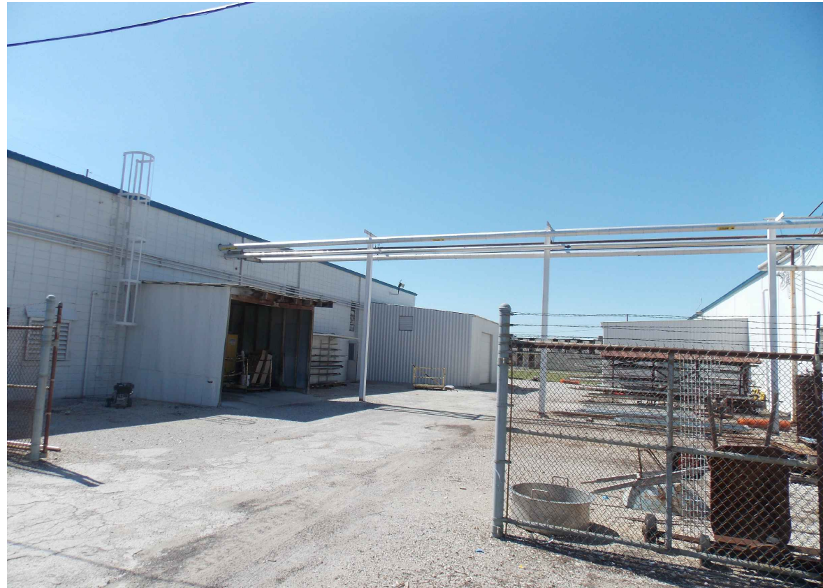
Photo L Existing Pipe Racks for Routing of 2" Nitrogen.
